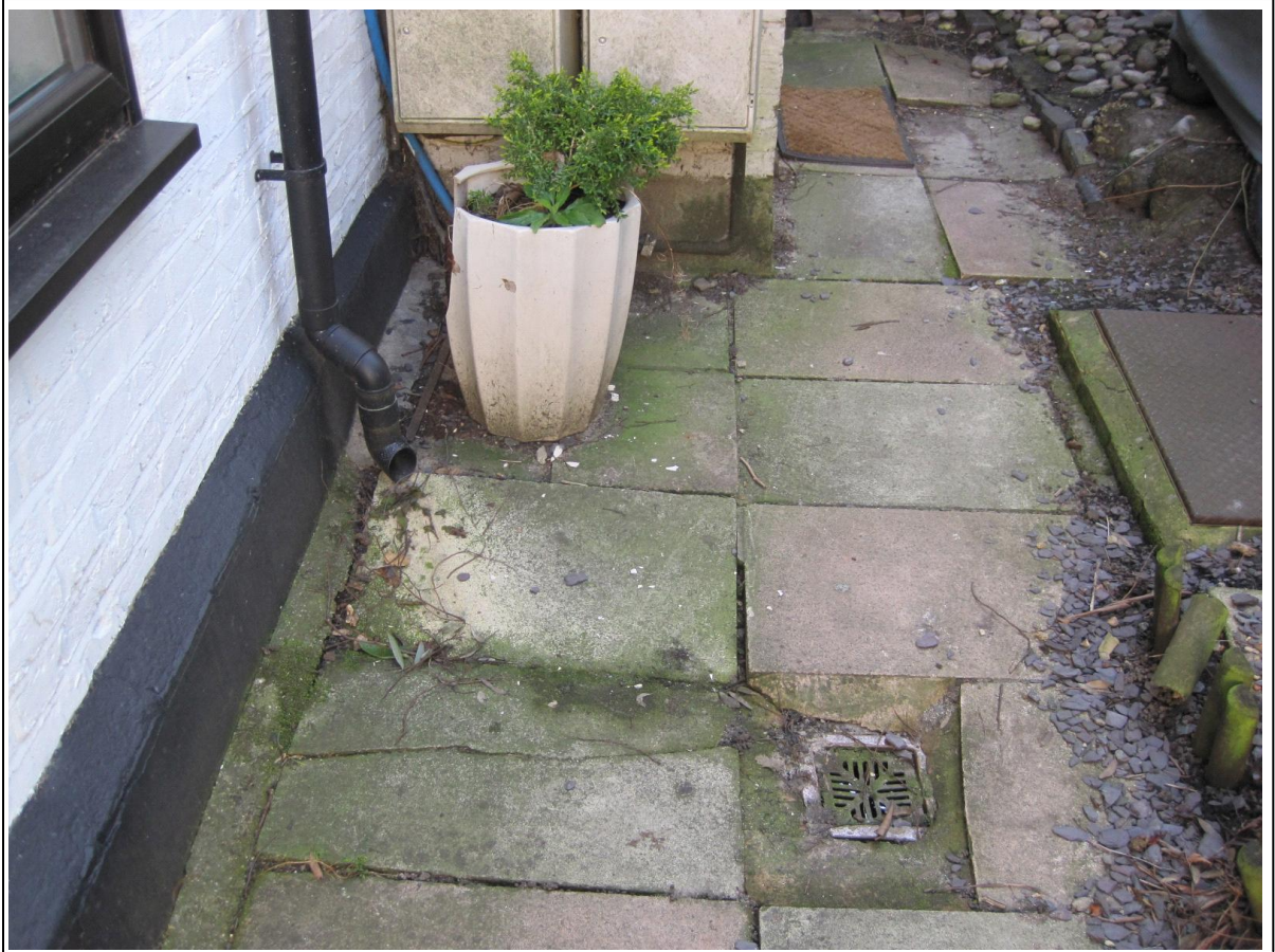
Uneven paving and discharge to remote gulley
