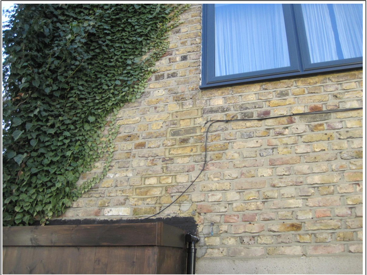
Re-pointing to front elevation
